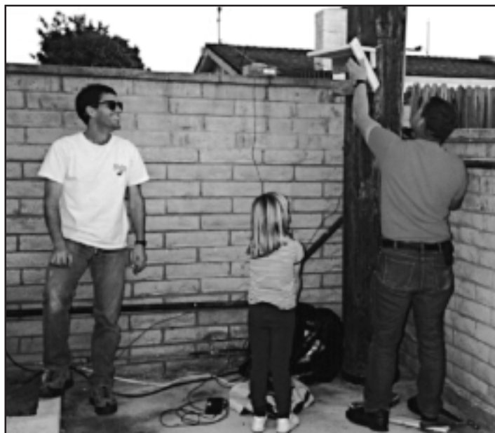
Local help. In La Puente, homeowner Joe Baeli, assisted by daughter Elizabeth, is constructing a stand to raise our GPS receiver. Aaron Martin of the Institute of Crustal Studies is also pictured.
